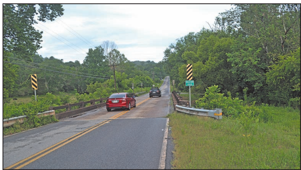
Brasstown Creek Bridge, or SR 66 Bridge, has been in service since 1940. A new bridge will soon be erected nearby to act as a replacement. Photo/Lowell Nicholson
